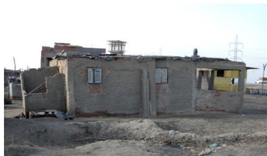
Fig (9) An example of an eroding reinforced concrete skeleton dwelling on the lake shores, which proves that building with concrete is not a sustainable nor climatic responsive approach.
