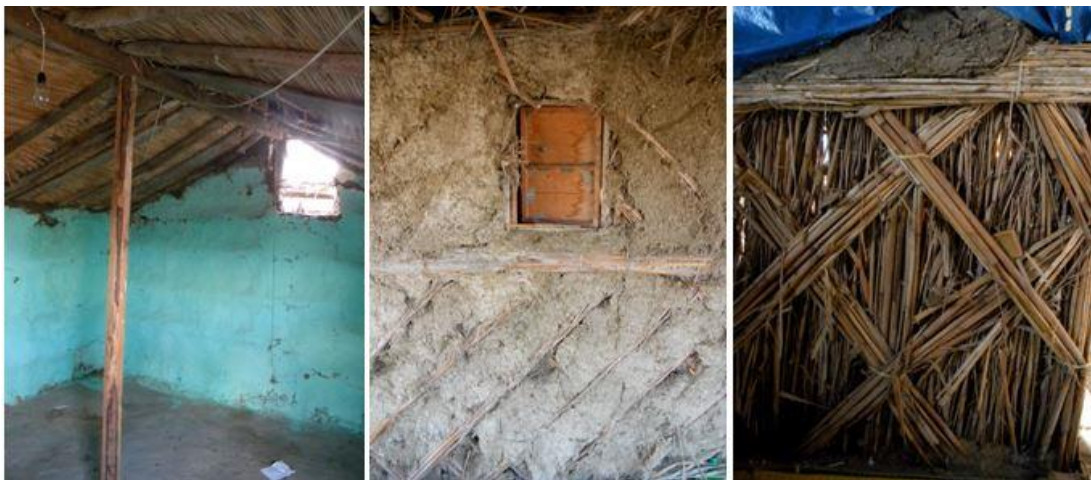
Fig (6) Showing the small openings, the structure of the reeds and the different textures and finishes applied.
