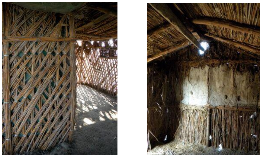
Fig (5) To the left an interior shot for the Al Aesh structure and to the right for Al Koshrk one.
