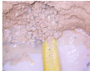
After: Drainage pipe
