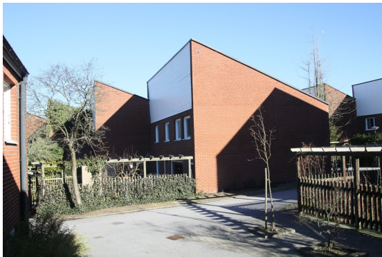
Fig. 2. View of the measurement area at street level, house 63.
