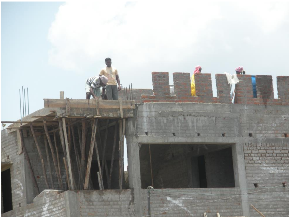
Figure 12: Picture from the construction site.
