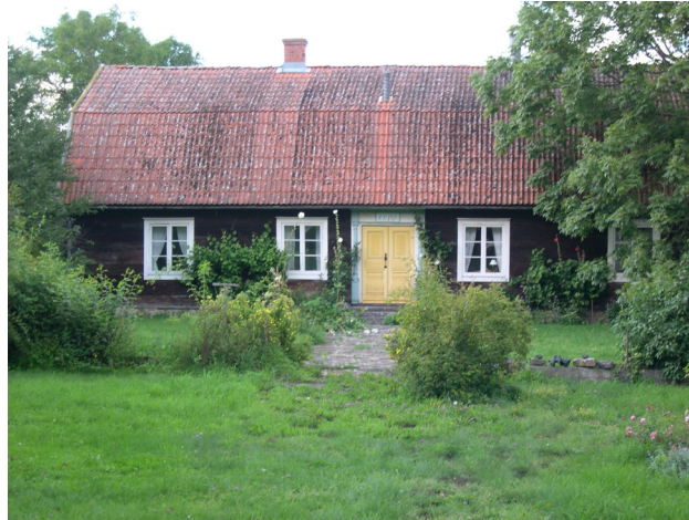
Fig. 3. This dwelling is from the beginning of the 19 th century with the wooden construction visible and tared. Together with the white windows and polychrome main entrance it's a typical local coloring at Öland during the period.
