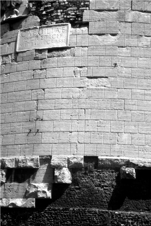
Fig. 25 (above). The tomb of Caecilia Metella. The travertine revetment of the drum. Photo by the author 2002.
