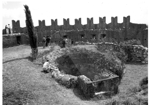
Fig. 35. The tomb of Caecilia Metella. The top of the drum with remains of a broken vault in the centre. Photo by N. Hillbom 1998.
