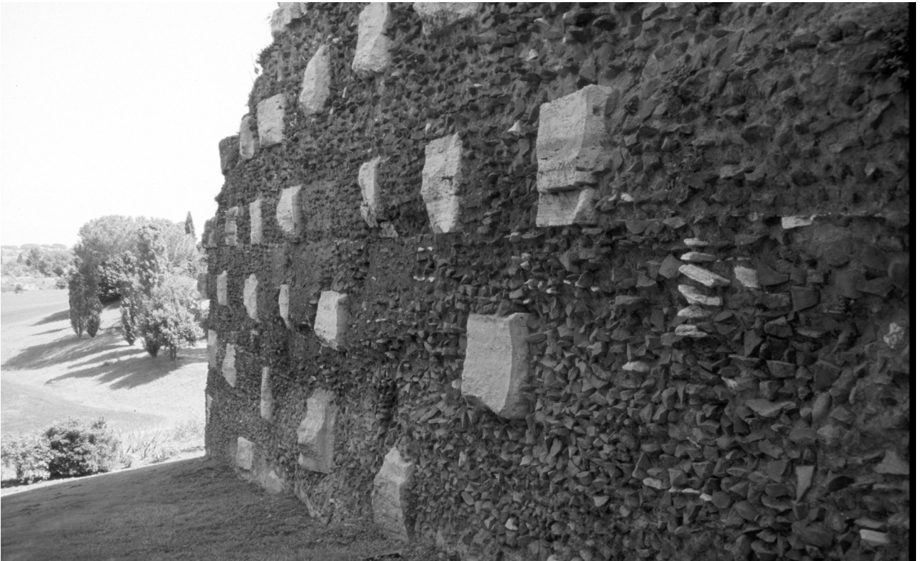
Fig. 13 (top right). The tomb of Caecilia Metella. The top layers of the podium and the base of the drum (SU20–23) on the west side of the monument. The lowest blocks (SU20) may have backed a protruding fascia . Photo by the author 2001.
