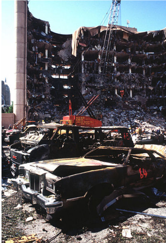
Figur 14 Murrah Federal Office Building i Oklahoma City efter bombattacken 1995 (Public Domain photo courtesy of the US Federal Government).
