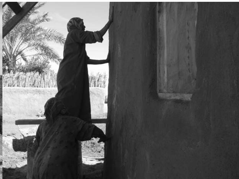
Ladies are always responsible for final mud rendering process for building facades.
