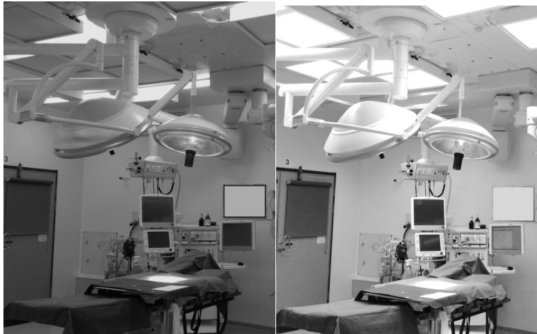
Figure 2. The existing general lighting (left) compared to the test general lighting (right).
