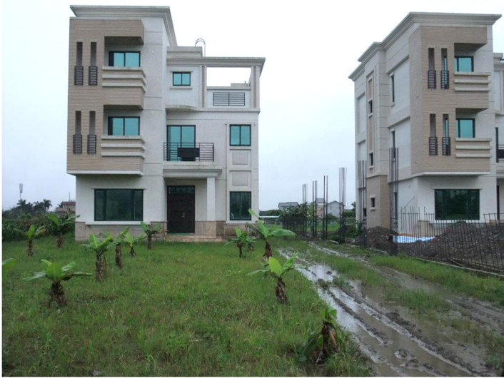
Photograph 1. Newly-built farmhouse in Ji-An, Hualien.
