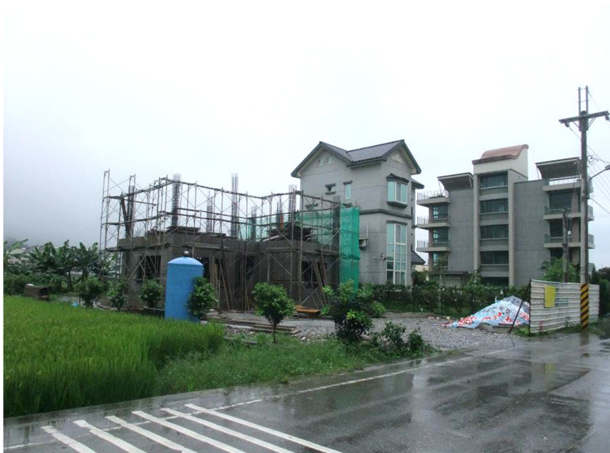
Photograph 5. Farmhouse under construction in Ji-An, Hualien
