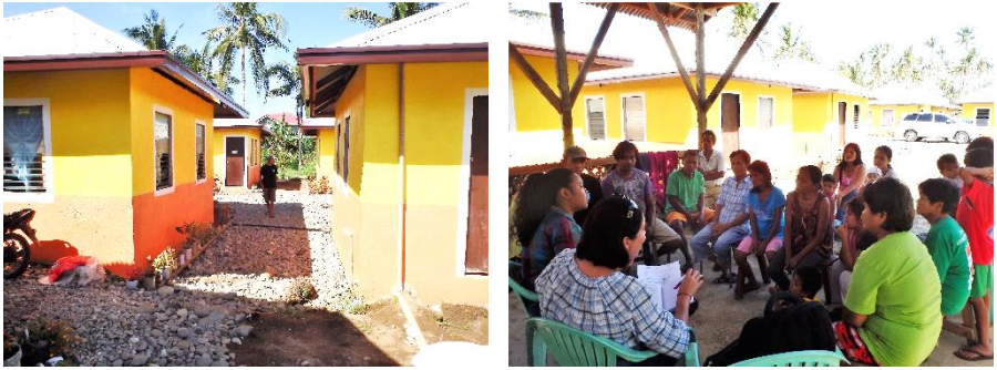
Figure 4.7 Community-driven reconstruction in relocated site by We Effect in Barangay Guintagbucan, Abuyog. Clustering of houses, focus group discussion with users. Pictures by the author, March 17, 2015
