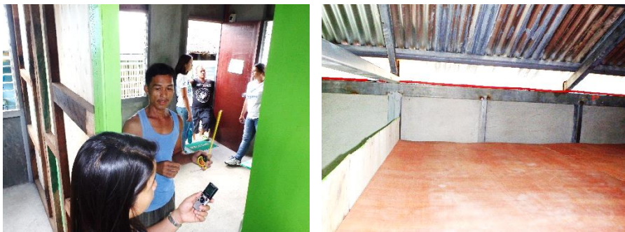
Figure 4.22 Housing solution with interior partitions and a loft for crawling self-built by the owner, Barangay Poblacion, Burauen. Pictures: by the author, March 13/2015
