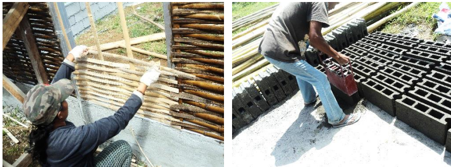
Figure 4.13 Woman weaving bamboo in a wall and man producing concrete hollow blocks, We Effect's pilot project in Barangay Dolores, Ormoc. Pictures: by the author, March 6, 2014
