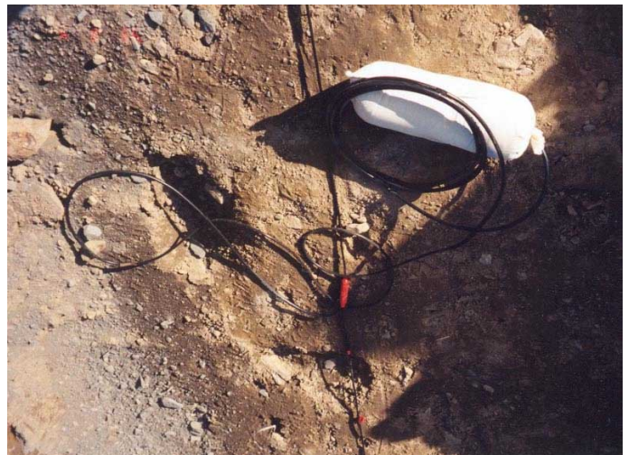
Figure 5. Installation of SP electrodes.
