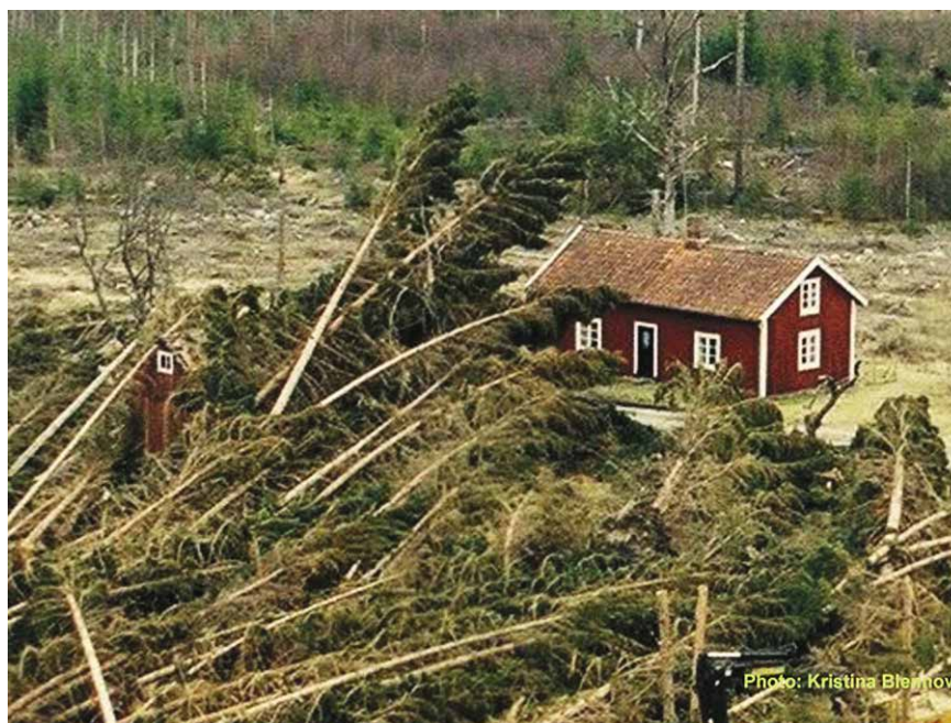
Figure 24. Wind damage after the storm Gudrun in southern Sweden on 8 January 2005. (Photo by Kristina Blennow)
