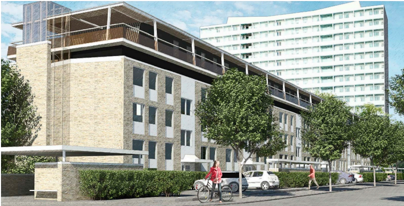
Figure 4.9 The proposed vertical extension for one of the buildings from case 4. Artwork courtesy of Jaenecke Arkitekter.
