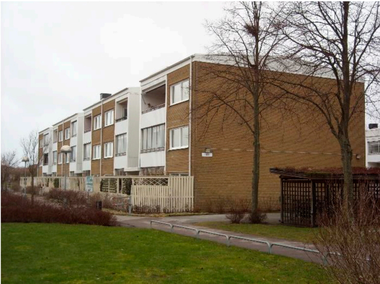
Figure 4.11 The low-rise building. Picture courtesy of Ahmed Hadzimuratovic and Marcus Swedmark.
