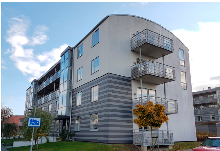
Figure 4.8 The realised renovation plus vertical extension of one of the buildings from case 3.
