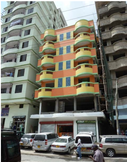
Fig. 8. Example showing newly built high-rise buildings in Kariakoo where the required side setbacks are not respected leading to poor ventilation inside the buildings.
