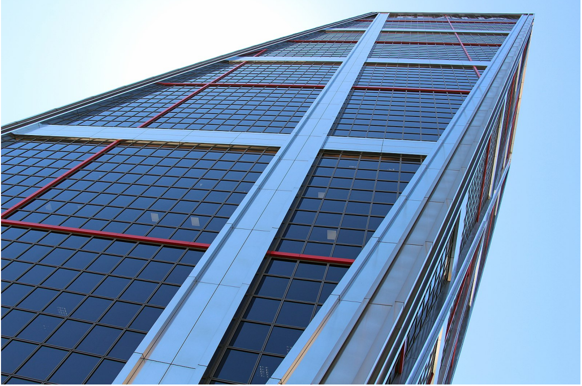
Figure 3.5: Close range observation of the Gates of Europe. The walls of the buildings are not ideally flat. The roughness effect has to be considered in channel generation.
