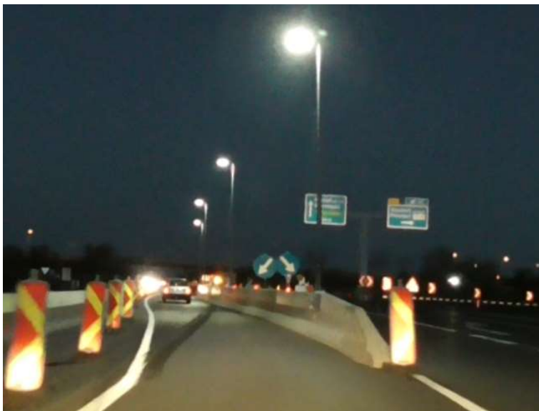
Figure 30: Illumination of critical zones
