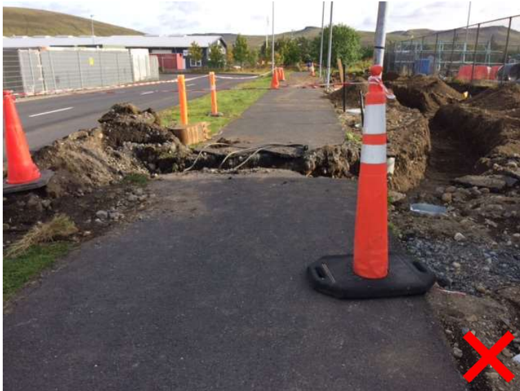
Figure 6: Works in the course of a bicycle path
