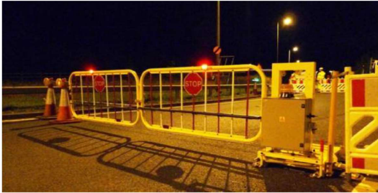
Figure 29: Automatic gate to control access to the airlock
