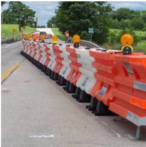
Figure 28: Water-filled portable vehicle restraint systems
