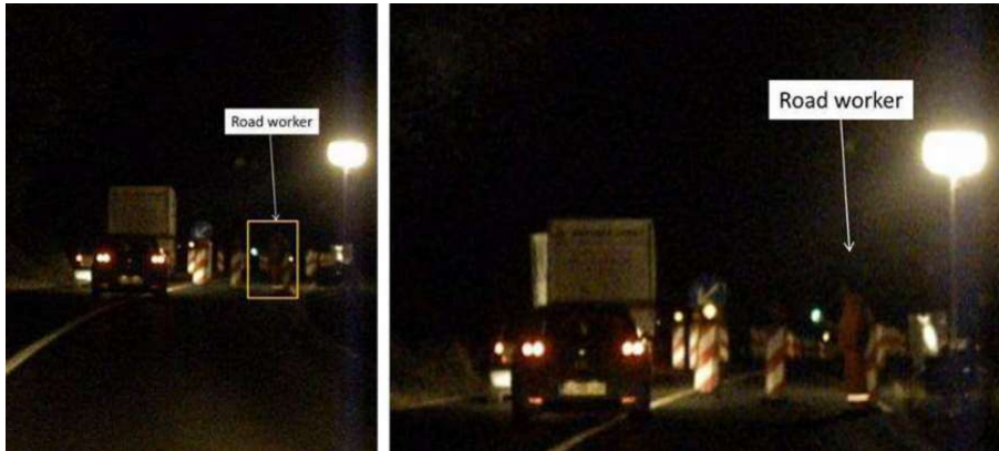
Figure 7: Inappropriate clothing of a worker at a work zone
