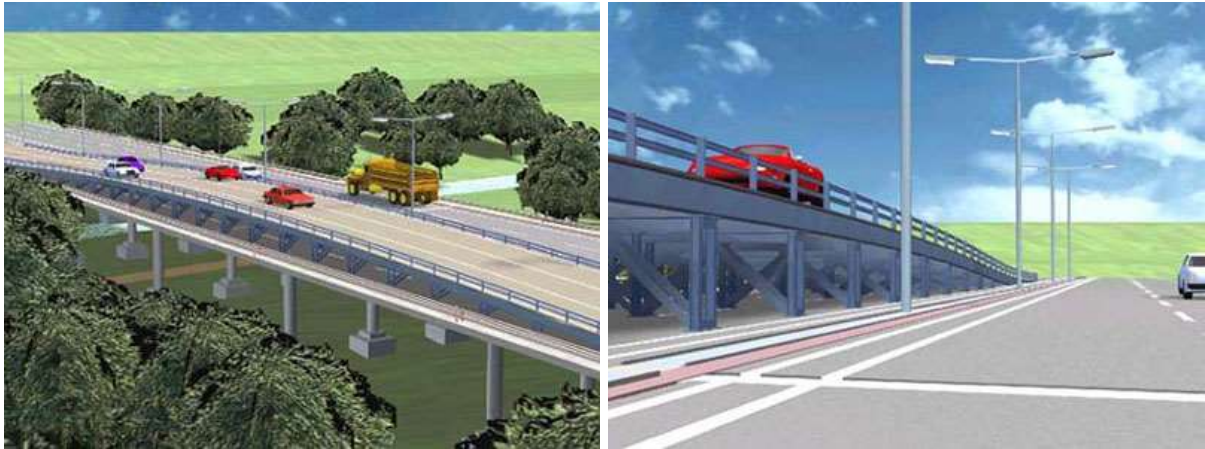
Figure 33: Temporary bridge (fly over)
