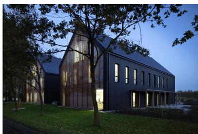
Figure 5. Photograph of the building, as built, taken from west facing towards east.
