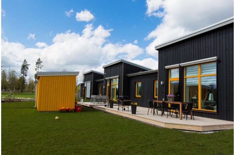
Figure 3.14 Photo of Solallén. Facade towards south
