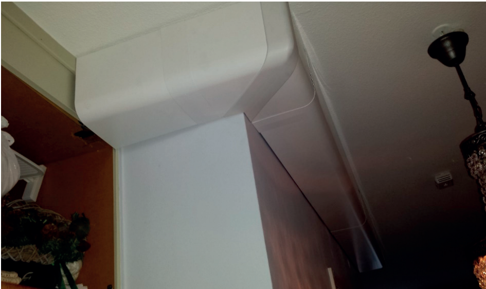
Figure A2.4: Picture of covered ducts inside apartments after installation.
