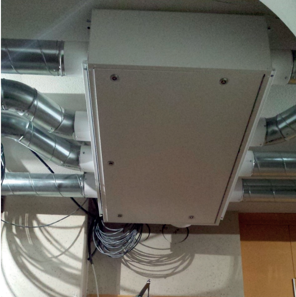
Figure A2.1: Picture of distribution box in hallway during installation.
