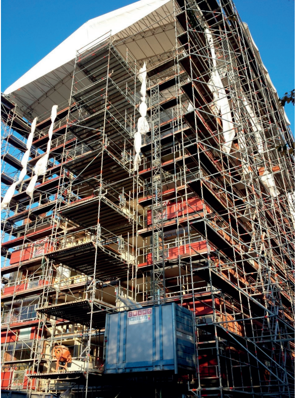
Figure A1.4: Example of weather protection during renovation.
