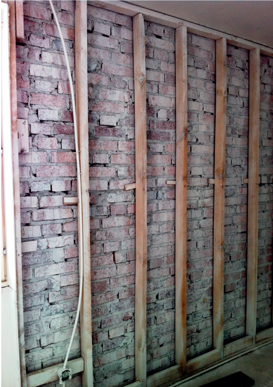
Figure A1.1: Exterior masonry wall in an apartment during renovation.
