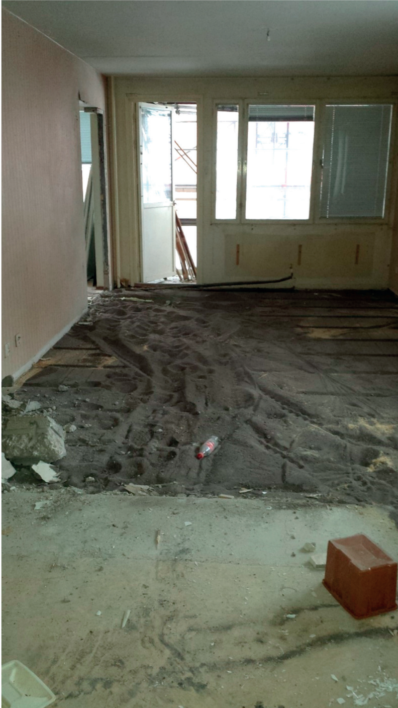
Figure A1.2: Beneath floorboards in living room during renovation.
