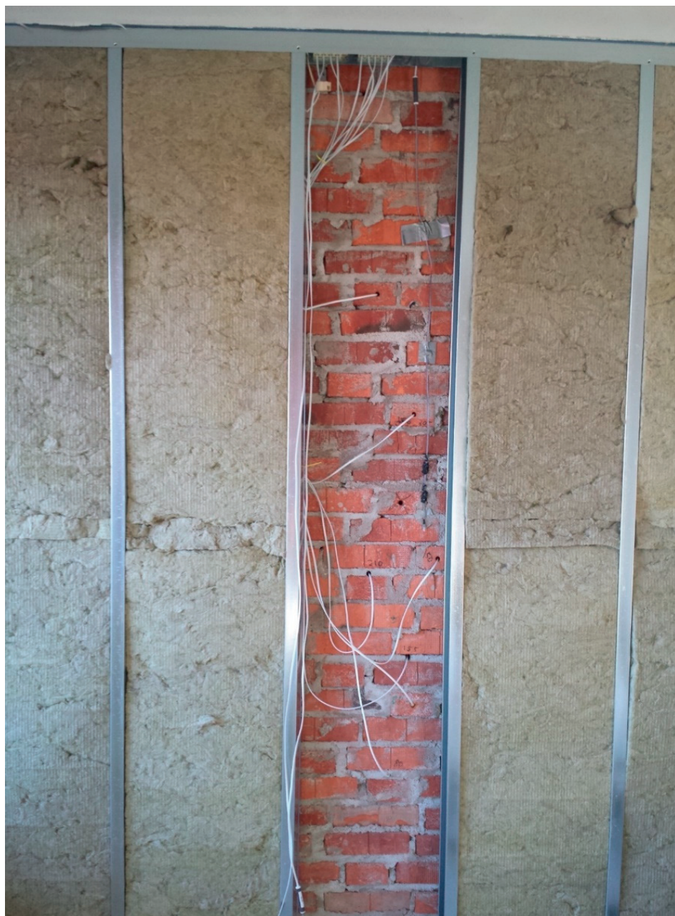
Figure A1.5: Sensor installation behind new internal insulation with steel studs.
