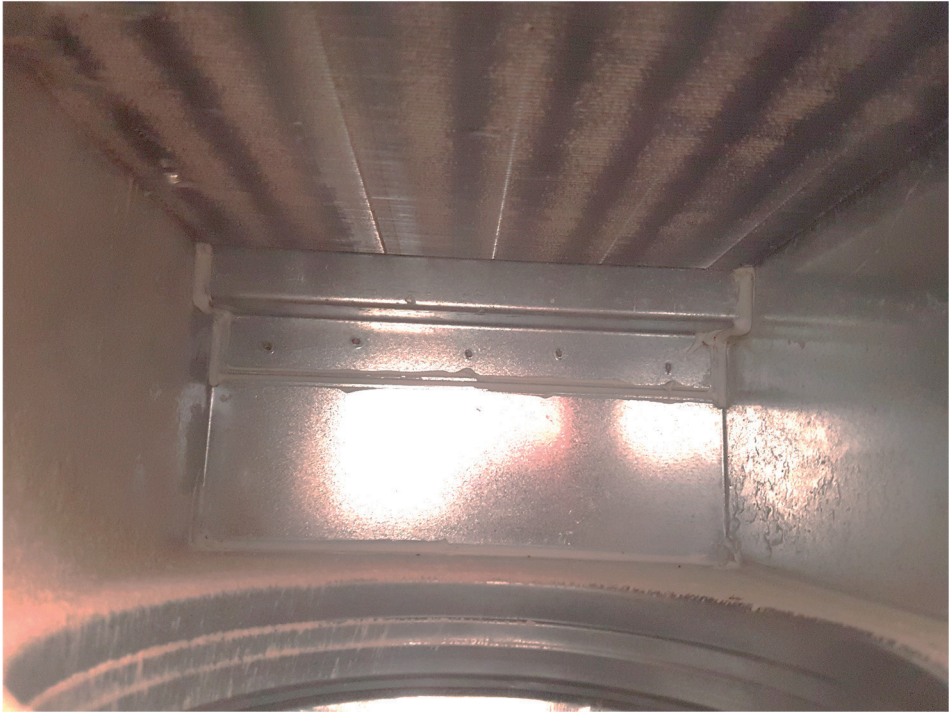
Figure A3.2: Contamination of heat exchanger in lab.
