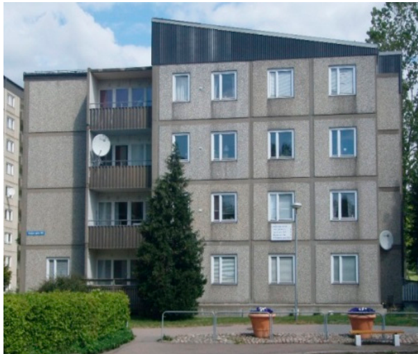
Figure 4.1 One of the buildings from case study 1.1 before renovation. Picture courtesy of Åke Blomsterberg.
