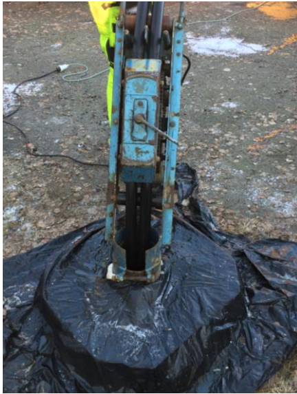
Figure 5 – Installation of single and double U-tube ground collectors in the 200-m deep borehole for in-situ tests.
