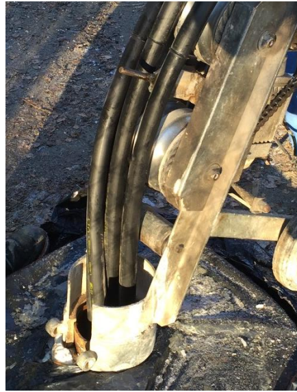
Figure 5 – Installation of single and double U-tube ground collectors in the 200-m deep borehole for in-situ tests.
