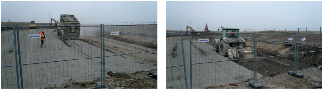
(a) Spreading out binder material.
