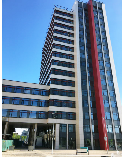
Figure 3: Example of a ventilated façade on a building in Riga, Latvia, (a) during construction with exposed insulation and railings (b) over the entire façade of a high rise building
