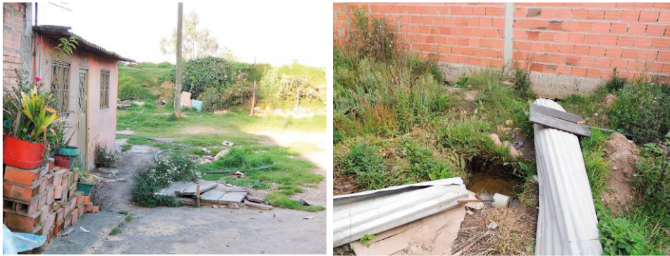
Figure 29. Wastewater disposal in San José I, Bosa
