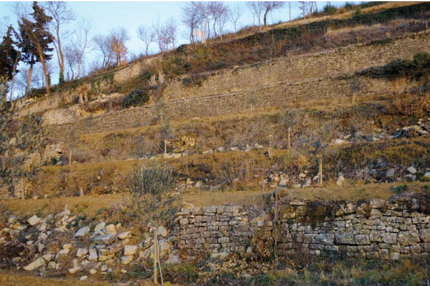
Figure 1: Dry stone retaining walls in Grožnjan (photo: Tanja Plešivčnik)
