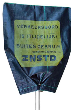
Figure 18. Covering restrictions when work shift is over.
