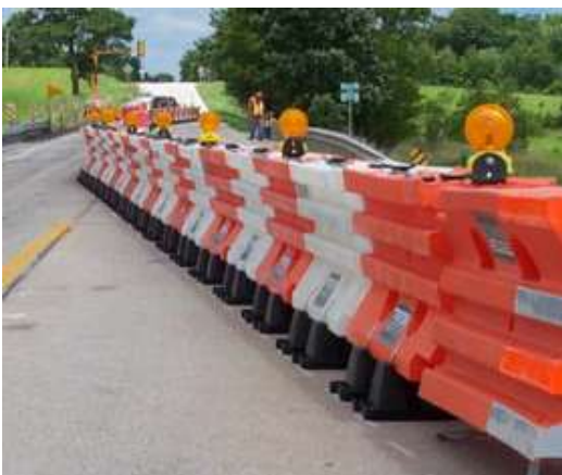
Figure 23. Water-filled portable vehicle restraint systems. Source: www.jtitraffic.com
