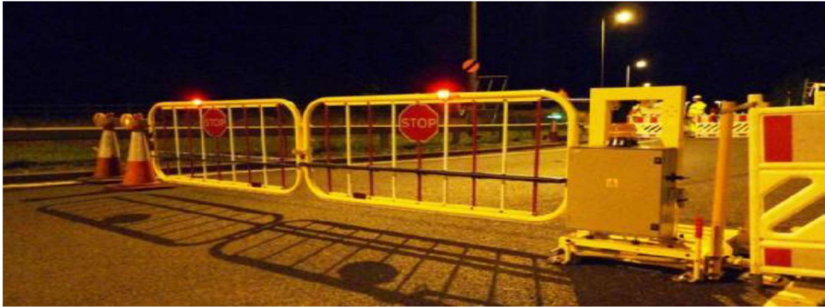
Figure 26. Automatic gate to control access to the airlock. Source: Highway Safety Hub http://www.highwayssafetyhub.com/roadworks-vehicle-incursions-2018.html
