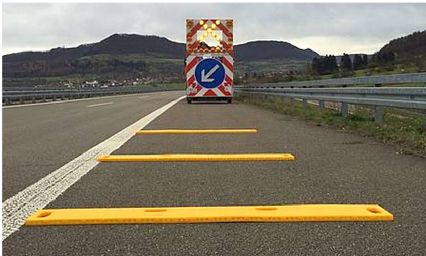
Figure 1516. Portable rumble strips on hard shoulder.
