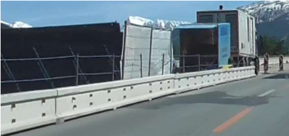
Figure 22. Small temporary vehicle restraint systems. Source: KfV
