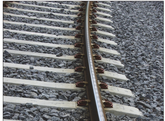
Figure 17. Overview of rail
