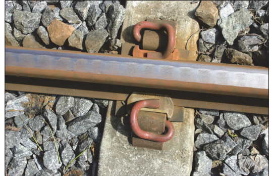
Figure 16. Detail of rail
