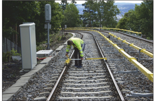
Figure 2. Preparing to measure rail corrugation.
