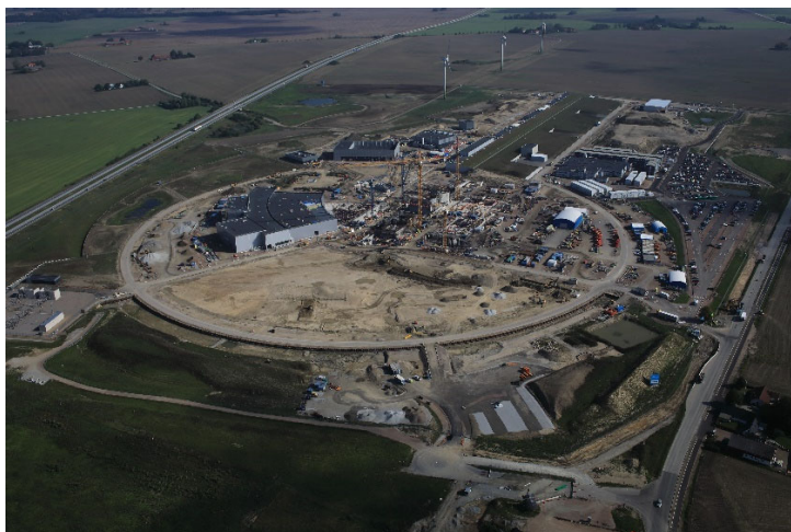
Figure 1. ESS construction site on September, 2018 [10].
