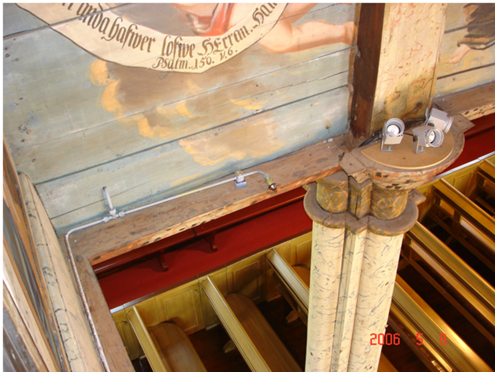
Figure 15 Sometimes, system piping cannot be concealed, but with the smaller diameter pipe associated with water mist fire protection systems, the installation can be made much less noticeable, as in Habo church. Photo: Magnus Arvidson.
