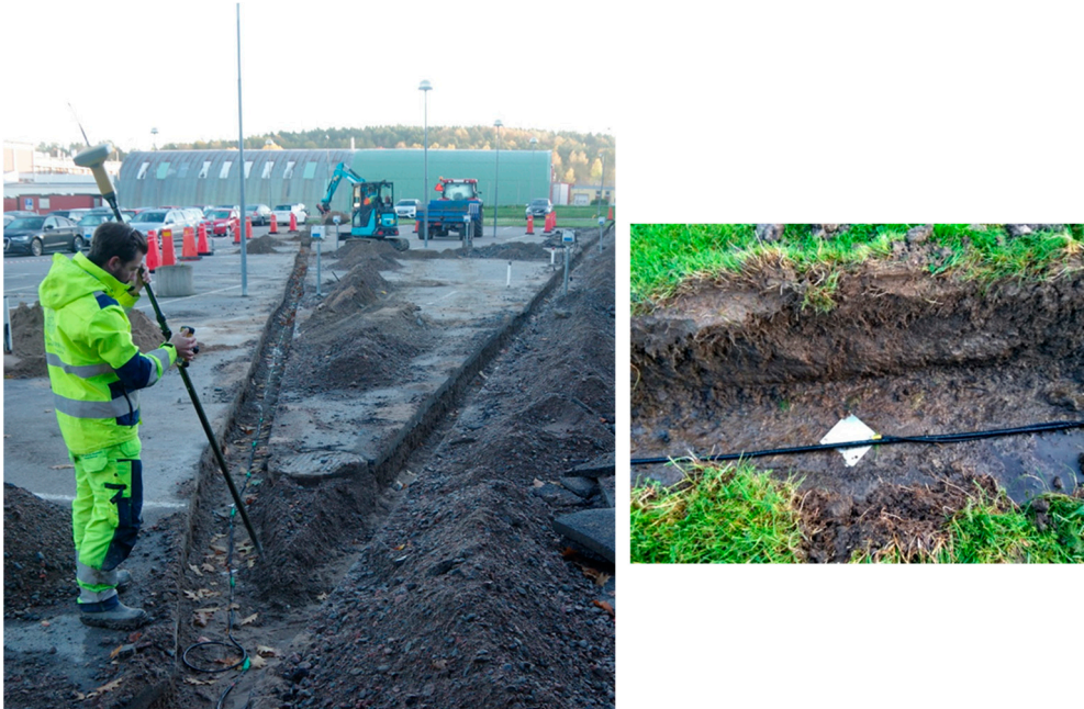
Figure 10. Permanent installation of electrodes for a DCIP monitoring experiment. Alingsås, Sweden.
