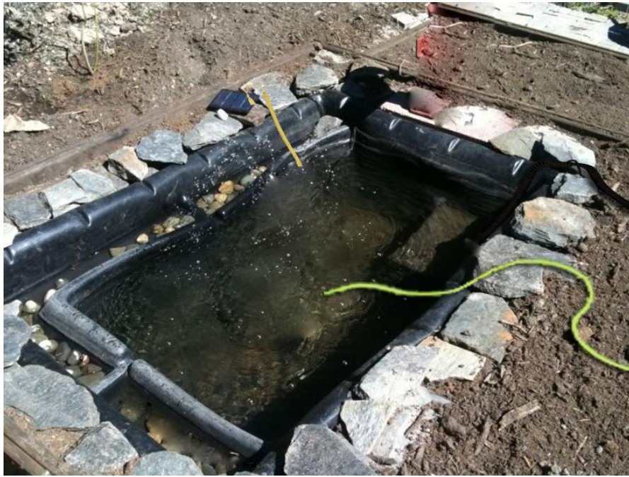
Fig. 3: Construction of experimental salt-gradient solar pond
