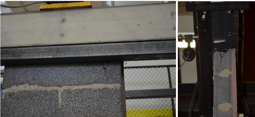
Figure LWA2_W11_1 Local crushing at the upper loading plate, at the corner.
