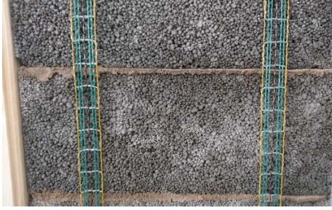
Figure 2.6 High strength steel wire strips before embedment in strengthening mortar.
