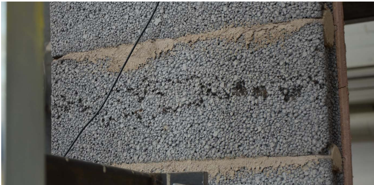
Figure 3.3 Flexural compressive failure in an LWA block wall.
