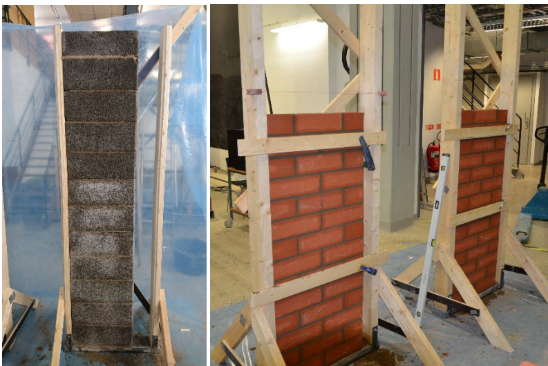
Figure 2.7 Manufacturing of the LWA block walls in series 2 (left); clay brick walls in series 3 (left).
