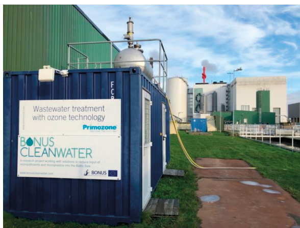
Figure 2. Photograph of the ozone pilot plant housed in a container located at the Lundåkra WWTP.
