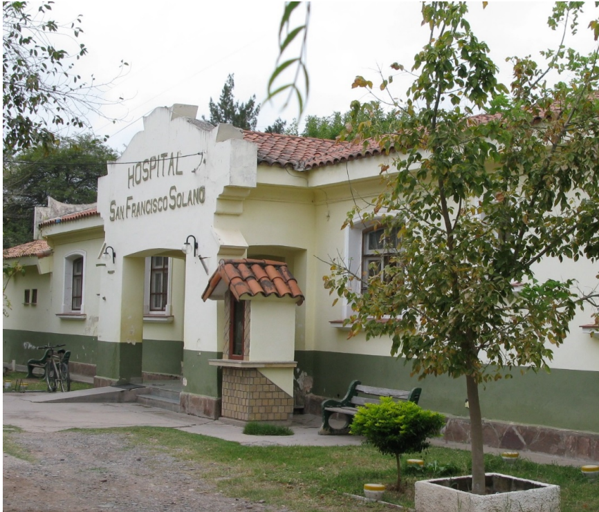
Figure 8: The hospital in El Galpon, Chaco area, Salta Province. Photo courtesy: Pia Tallving.
