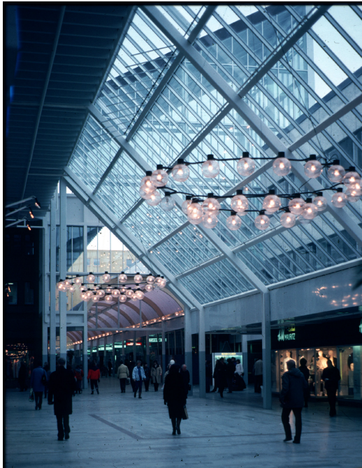
Figure 1.12 Skärholmen Centre, Stockholm. Glazing constructed in 1984.
