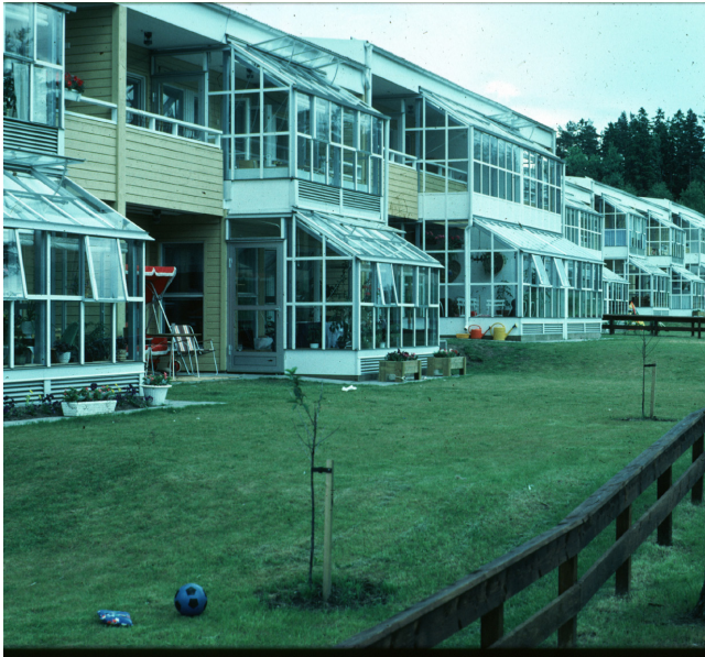
Figure 1.15 Blocks of flats with glazed verandas, Taberg, 1981.
