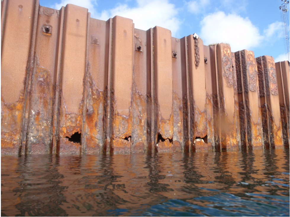
Figure 4 Typical corrosion pattern in the water line on a sheet pile wall. The backfill is visible through the holes in the piles.
