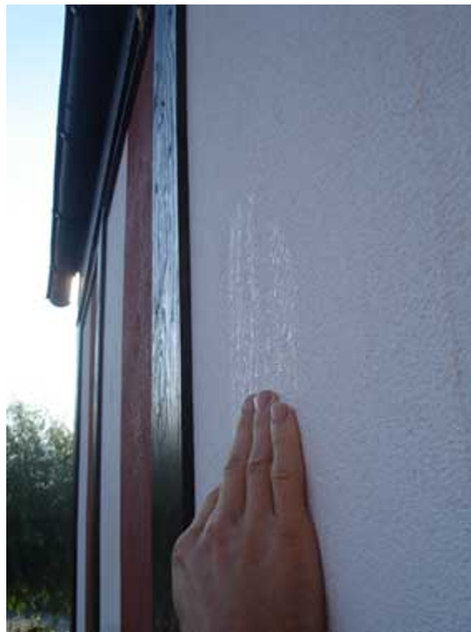
Figure 2.11: Night condensation of a north-facing wall on the test house (Paper III) around 8 in the morning in October 2007. No condensation was found on the south-facing façades or on the walls with render on bricks.
