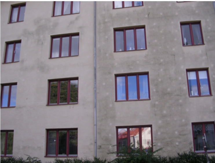
Figure 2.7: A façade that shows white spots.
