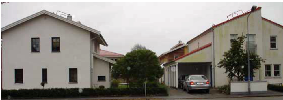
Figure 2.3: Two neighboring houses in southernmost part of Sweden. The house to the left has no discolorations whereas the house to the right have pronounced discolorations due to algae growth.
