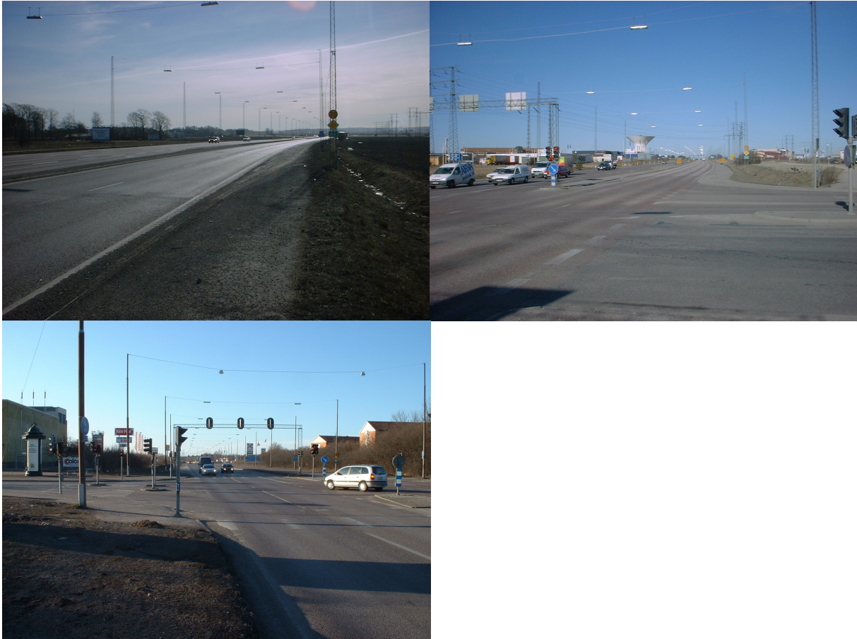
Figure 35 a-c European Highway E4 in outer part of Uppsala coming from Rural area (upper left, U14), shifting slightly to a more urban form with signalised intersections (upper right, U17) and being transformed to an urban four lane street (lower left, U23)
