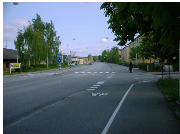
Figure 13 Separated bicycle facility crosses intersecting minor street (left and right)
