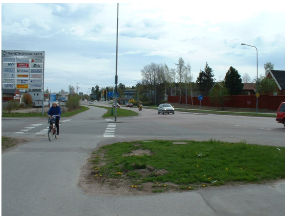
Figure 13 Separated bicycle facility crosses intersecting minor street (left and right)
