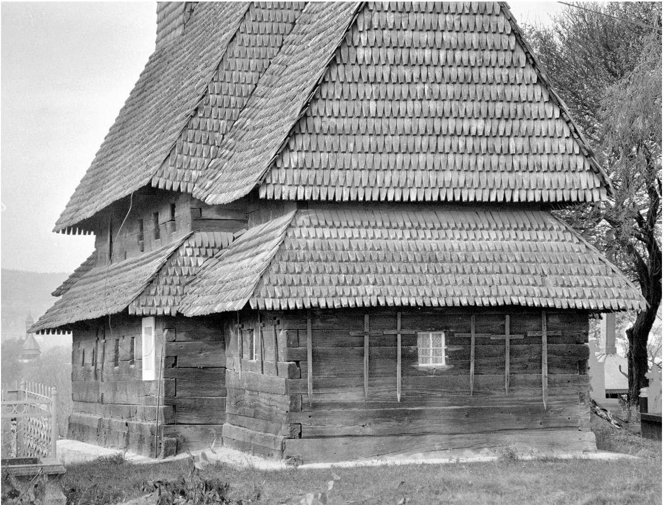
45 Apșa de Mijloc Susani . This medium sized wooden church, from the first decade of the 18th century, was excellently built with well levelled walls and flush covert joints. Photo: October 2000.
