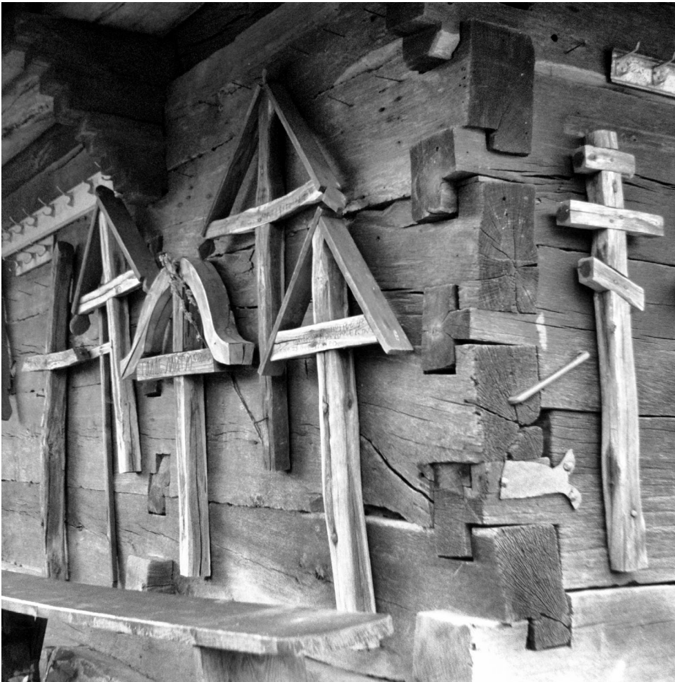
52 Steblivka . In the construction of this church the master carpenter shifted here and there from the common tabled joints to double tabled joints. Photo: July 1994.
