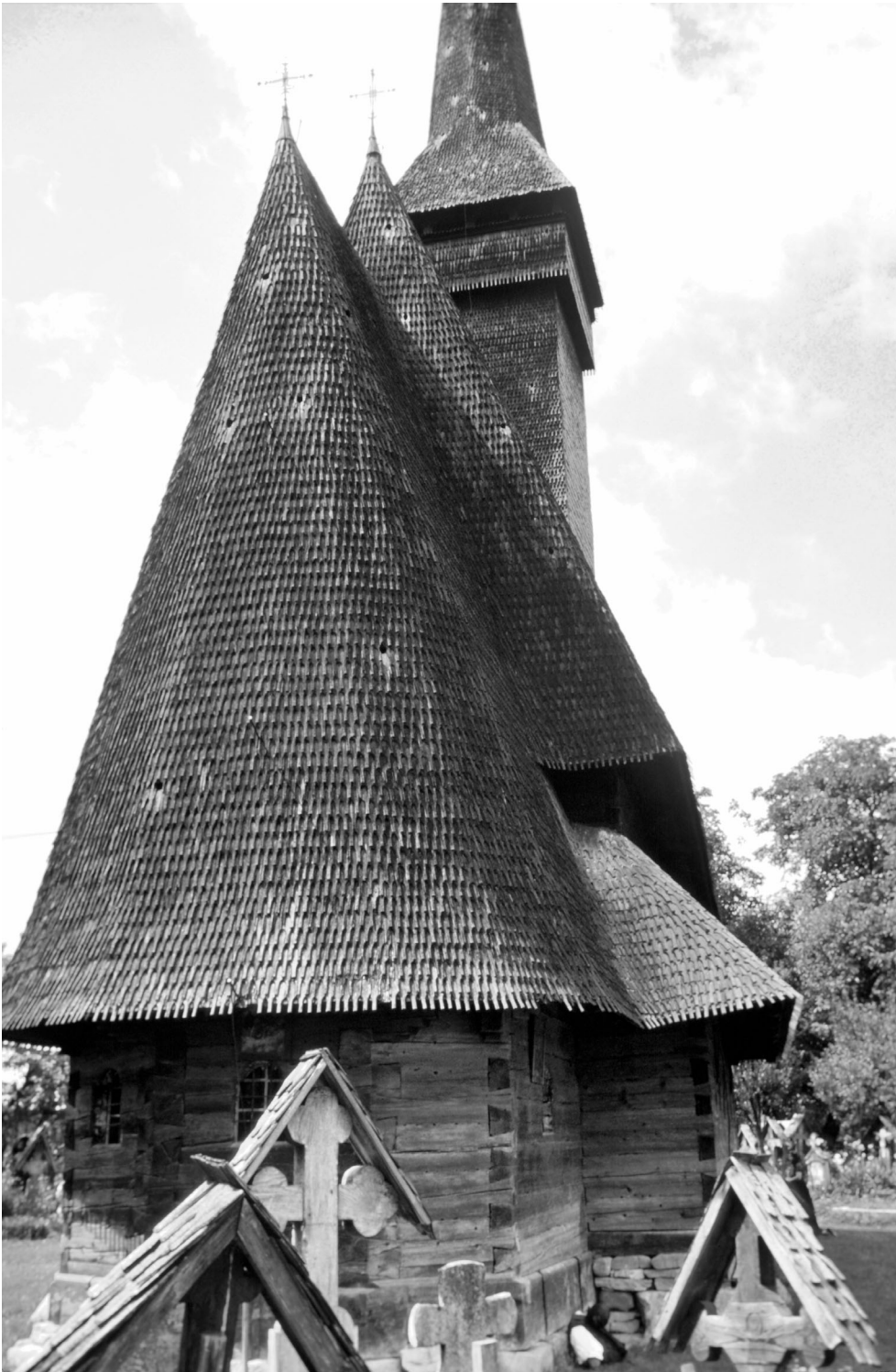
82 Ieud Șes . This church, particularly known as the wooden cathedral of Maramureș, built probably in the 1710s or in the previous decades, retains the steepest roof of all known in the region. The rafters over the sanctuary might measure two times the width of the sanctuary or more. Photo: July 1993.
