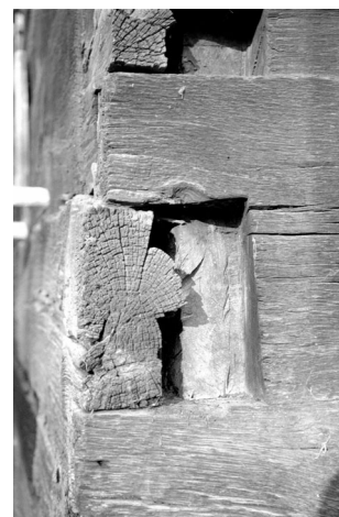
48 Breb . Settings in the north-western corner of the building damaged the hook in the picture exposing the covert cog. However, the damage was limited thanks to the presence of the heart of the tree in the hook. The visible traces indicate the cog was cut with an axe. Photo: October 2000.
