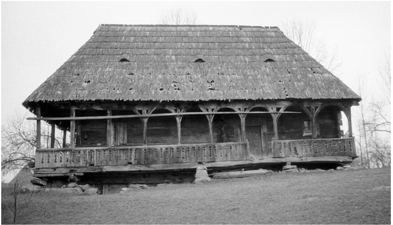
29 Sârbi. The manor house of the noble Dunca de Sârbi family (1690s). The corner joints present a small recess in the neck to improve the interlocking of the beams (below, left). Due to the limited length of the massive logs the house was extended lengthwise by posts, one of them also used as the left jamb of the entrance (below, right). Photos: March 1995, on the initial site (above and below), and August 1997, during its reconstruction in the Maramureș Museum.
