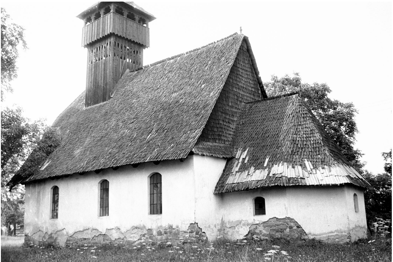
234 Sarasău . The sole medieval church of stone from an Easter community survives in Sarasău. However, the windows were enlarged and the tower rebuilt during comprehensive renovations in 1937. Photo: July 1994.
