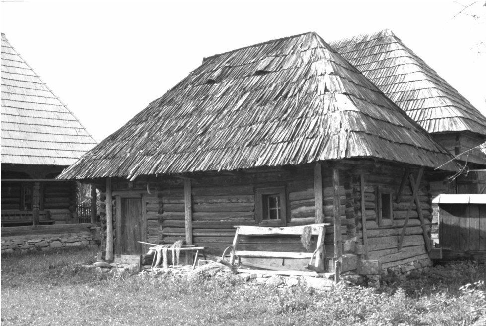
34 Ieud . Saved in a local private museum, the house of Moldovan Palaga Babii illustrates some of the simplest and oldest types of log houses, with only a small room and a dark ante-room, without any closed porch. However, considering the type of flush corner joints, the house can not be older than 100-150 years. Photo: September 2001.
