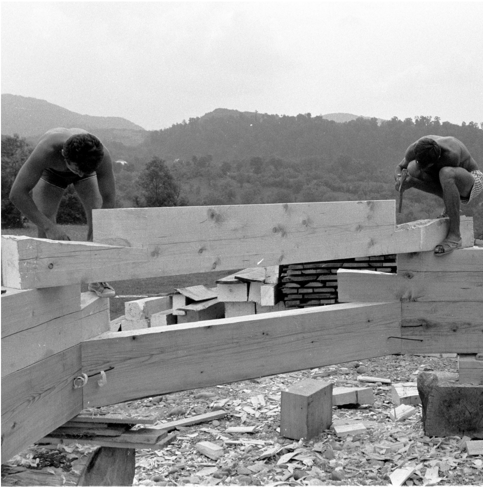
39 The Ethnographic Museum of Maramureș, Sighet-Dobăieș. The log building is still common in Southern Maramureș. During the last decade even some new wooden churches with traditional appearance were made. In this picture the carpenters worked with a wooden church for a Romanian community in Caracas, Venezuela. Photo: July 1994.
