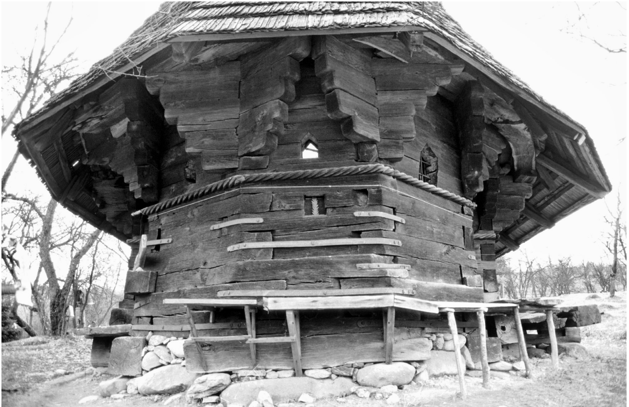
175 Sârbi Susani. The rear of the sanctuary with the joyful play of consoles under the eaves. The only original window seems to have been the square one below the moulding rope. The rope appears to have separated the earthly world from the heavenly one. Photo: Spring 1995.
