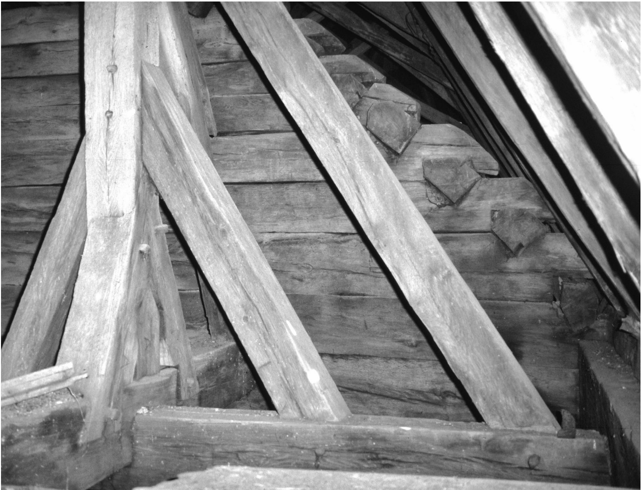
127 Apșa din Jos . The anchoring of the south-eastern upright in the massive transoms of the base. The transoms were interlocked with the lateral walls while the log fabric was still in construction assuring a stable connection between them. Photo: October 2000.
