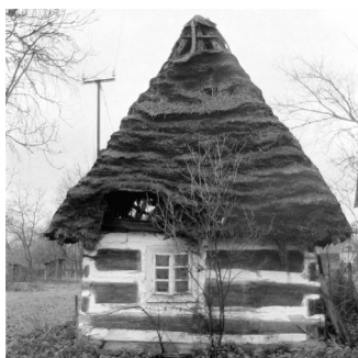
85 Tereblia. In some villages from the lowlands of Northern Maramureș it is still possible to observe ruinous thatched houses as this one of Hrulia Vasilina from Tereblia, probably erected in the 19th century. In this part of Maramureș the strips of daub sealing the walls are specifically emphasised in colours like white and blue. The low opening in the roof allowed the smoke to come out. Photo: November 2002.
