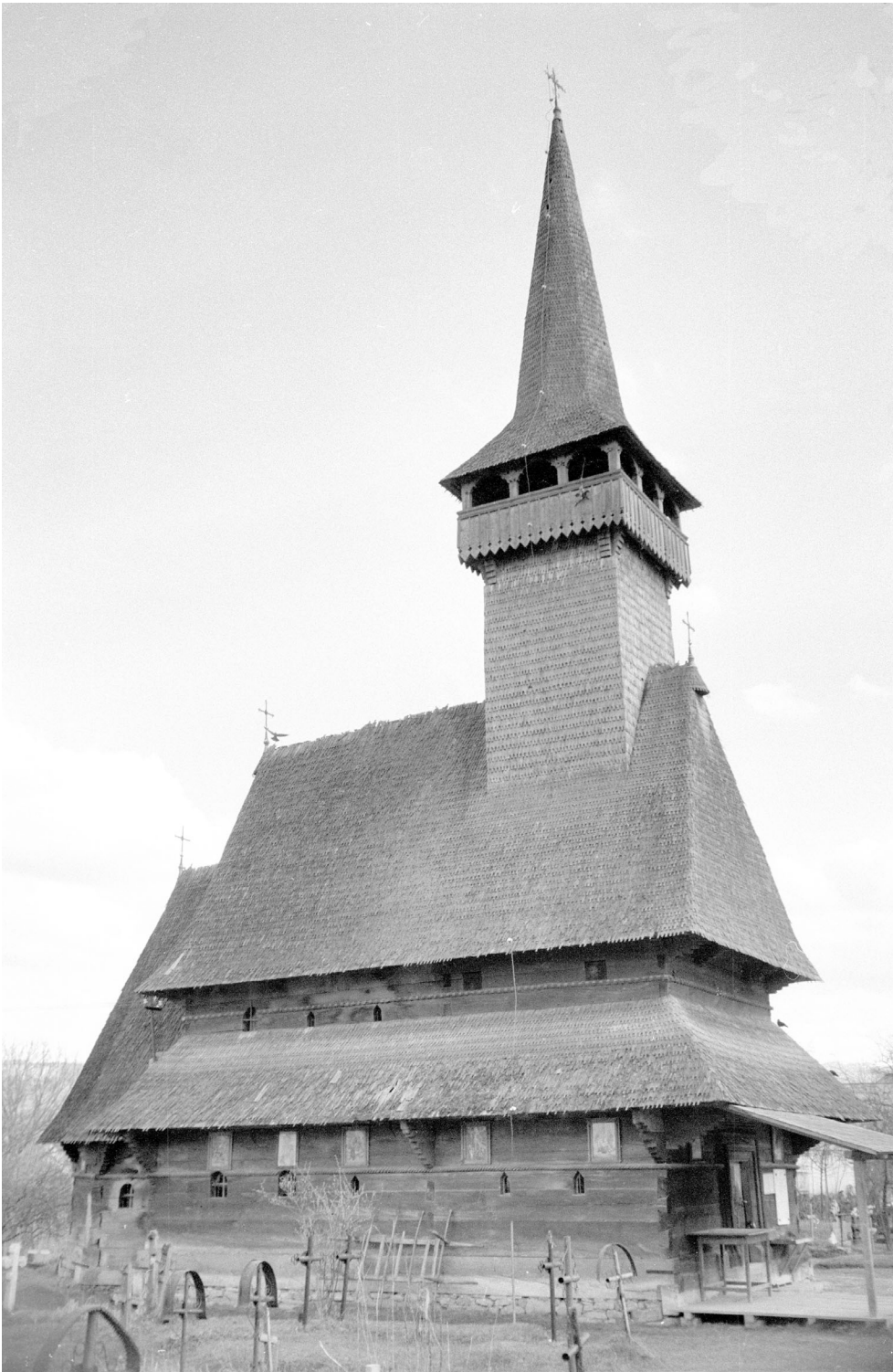
192 Sat Șugătag . The church is preserved in good condition. One of the specific features is the mouldings surrounding the log fabric on two levels, above both rows of windows. Wherever the horizontal mouldings appear they are cut above apertures indicating a symbolical distinction between the earthly world and the one above. Photo: April 1994.
