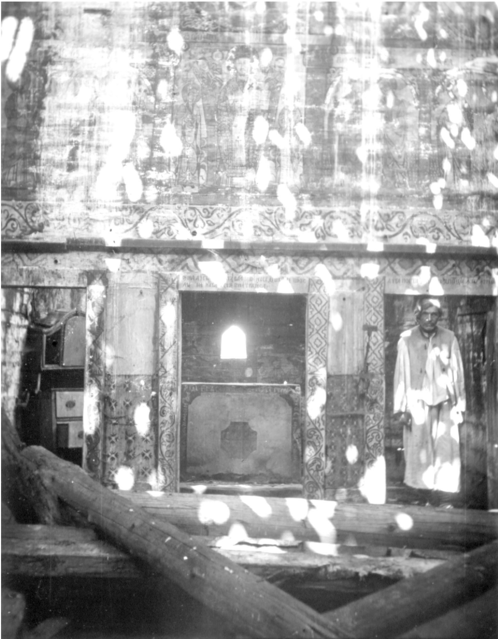
8 Berbești. Photo by Atanasie Popa, July 1932, just before its demolition (MIT, Arhiva CMIT, C3:4778). The picture was taken from inside the nave looking towards the sanctuary. The spots of light on the iconostasis and the timbers lying on the floor indicate the roof was in a poor state and the vault had fallen in.
