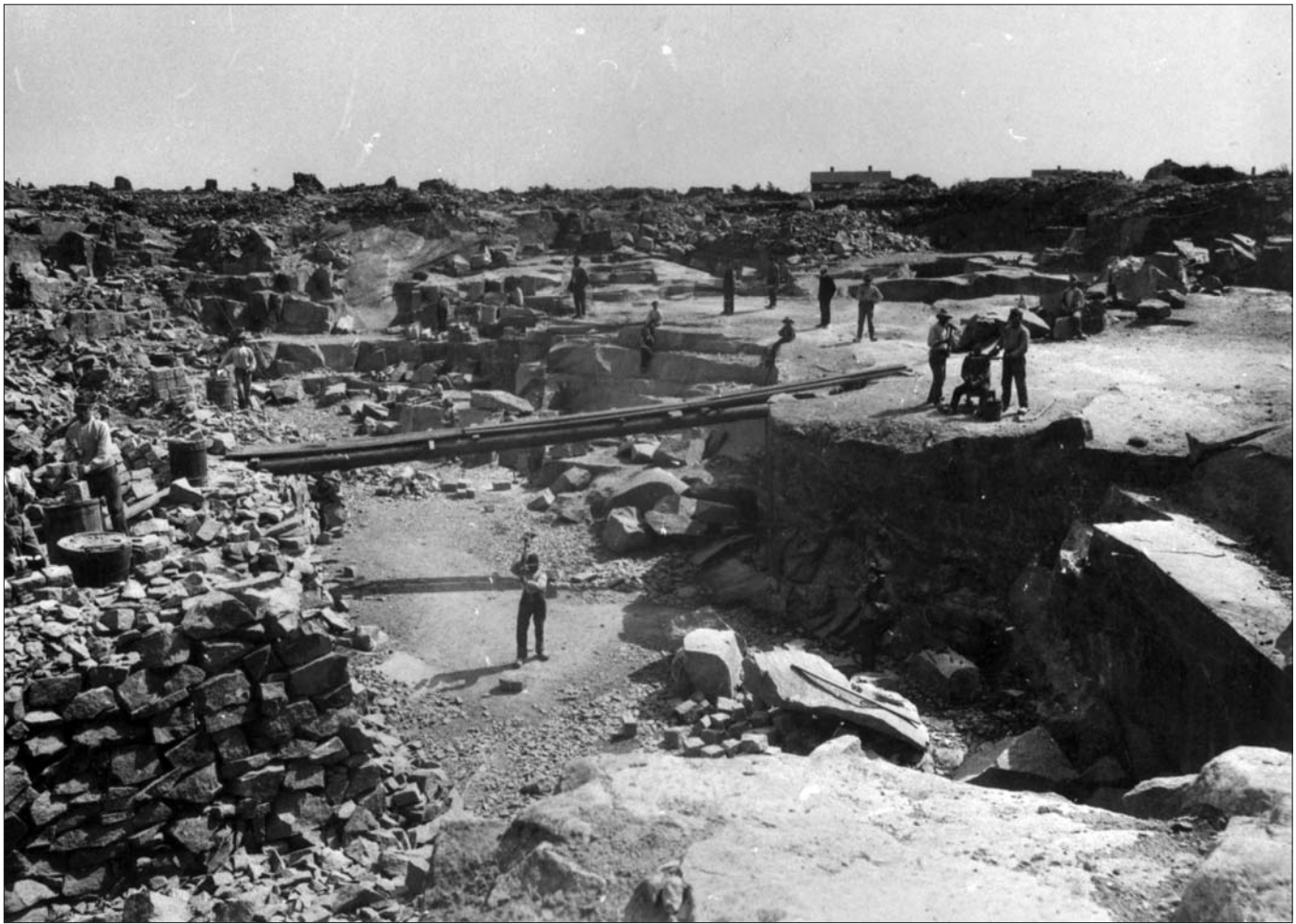
FIGURE 2. The Herrgård quarry on the island of Tjurkö in Blekinge. The photograph, probably taken about 1890, shows how thirty years of quarrying have rearranged the previously forested island. The picture manages to capture all stages of paving stone manufacture. In the upper right-hand corner we see a drilling team at work. One man is holding the drill while two others hit it with their sledgehammers. Down in the quarry pit a stonecutter is about to split a block into two paving stones. A man in the dump heap to the left is removing bumps from the side of a paving stone with a hammer and chisel. Behind him another trimmer is standing at his workstation and next to him is a pile of paving stones ready to be measured. Photo: Hjalmar Falk, Blekinge Museum.
