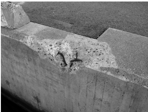
Figure 8. Local damage with corroding reinforcement.
