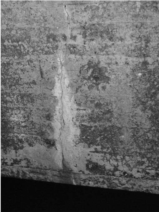
Figure 7. Typical vertical crack with signs of leaching calcium.
