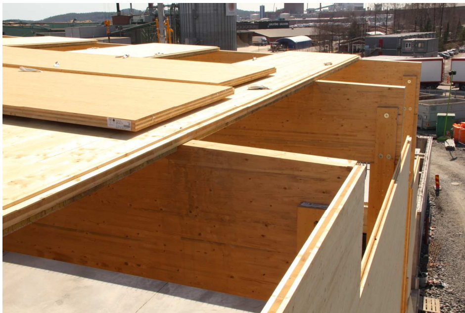
(b) A close-up picture of the CLT-decking.
