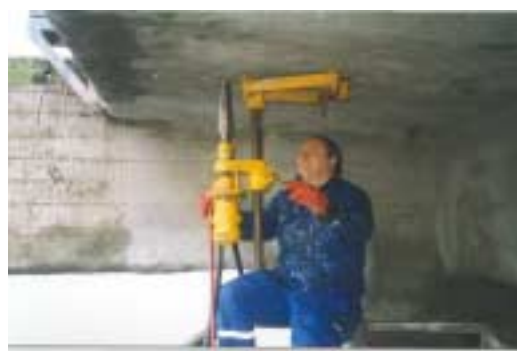
Figure 8: Installation of corrosion sensors in Norwegian quays, see also Figure 7.
