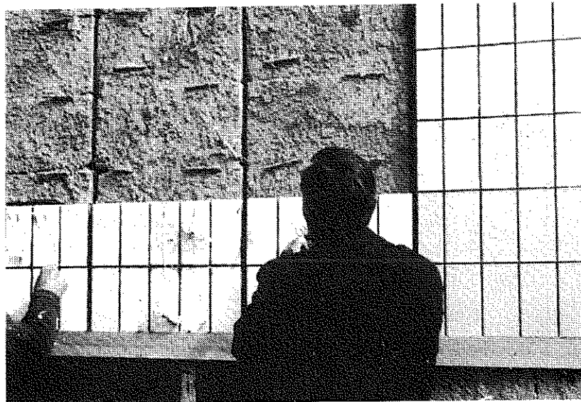
Figure 1.3.2q. Tile fixing, House I, south wall. Observe the special anchors for the fixing mortar. All wall elements in House I to be observed by strain-gauges etc were provided with these anchors while rest of the wall surfaces were provided with a normal net. The two vertical slots on each wall are holes intended for the moisture observations by use of wedge-shaped test specimens
