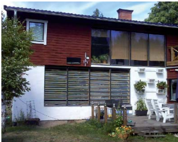
Figure 1.7 Parts of the south side showing the heavily glazed façade.
