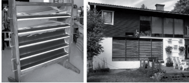
Fig. 2. Left: the prototype solar window. Right: the solar window in Solgården with closed reflectors.
