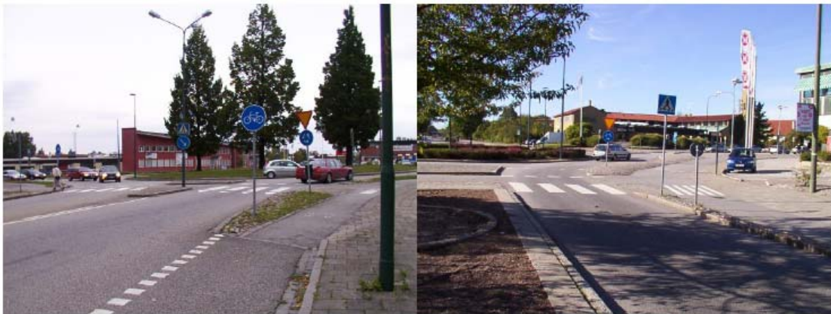
FIGURE 17 Roundabouts with different location of the yielding sign and line, Salleruppsvägen/Scheelegatan and Köpenhamnsvägen/Erikslustvägen, Malmö City
