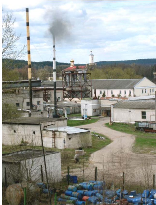
Industrial site in South-western Belarus
