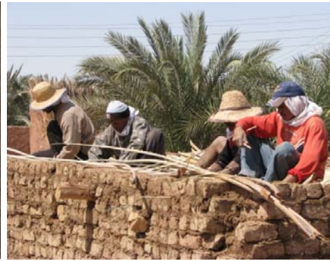
Figure 5.28 Placing palm leaves on top of reeds.
