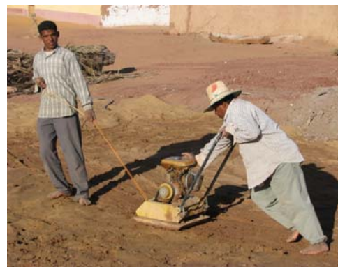
Figure 5.18 The site during soil replacement and compaction.
