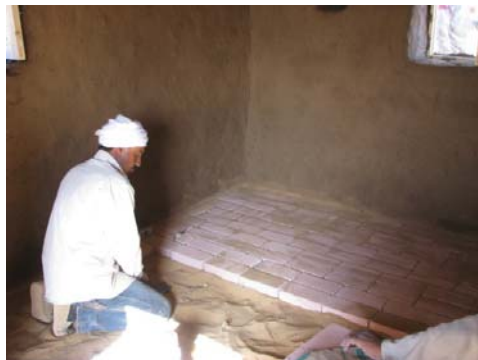
Figure 5.34 Floor making using sand tiles.
