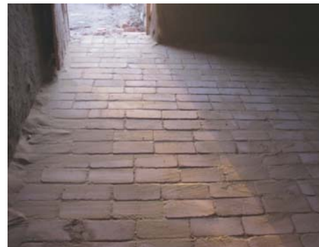
Figure 5.35 Sand floor tiles after finishing.
