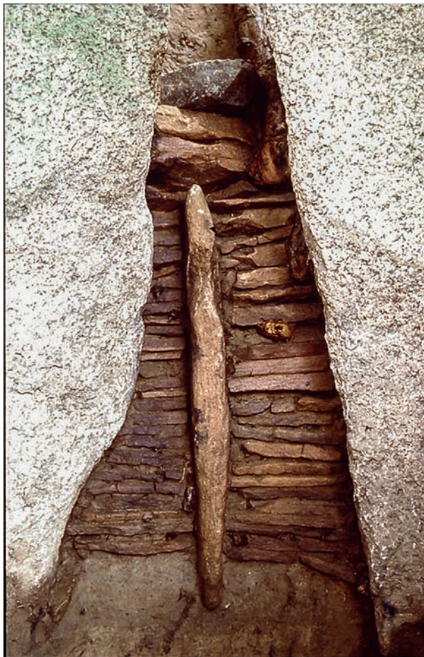
Fig. 1. A dry stone wall in the Hallebrøndshøj passage grave on Bornholm, Denmark. Photo: Svend Illum Hansen.
