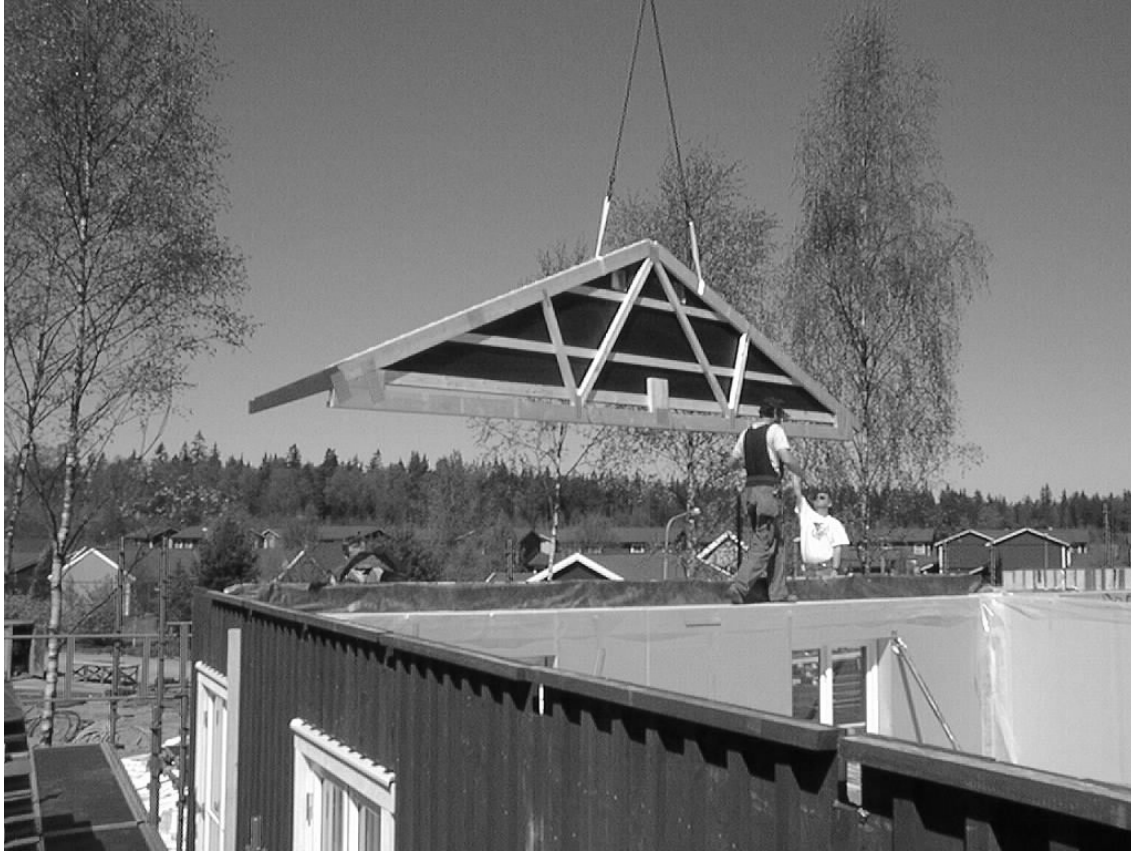
Figure 40: Construction element with attachments to facilitate unloading.
